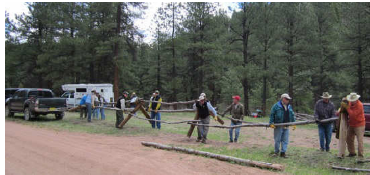
Moving the Old Buck & Pole Fence
