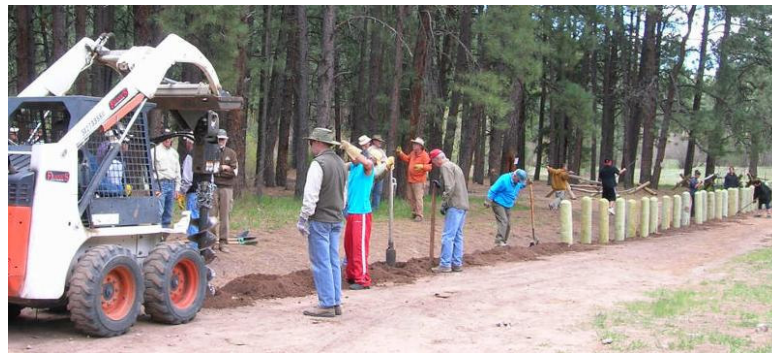
Drilling and Digging
