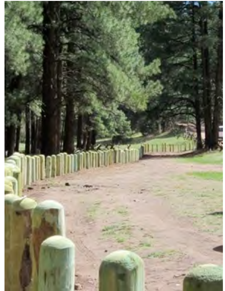
Completed project after a productive day's work
